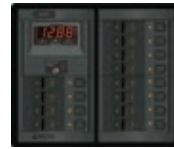
BRANCH C/B WITH DIGITAL METER
